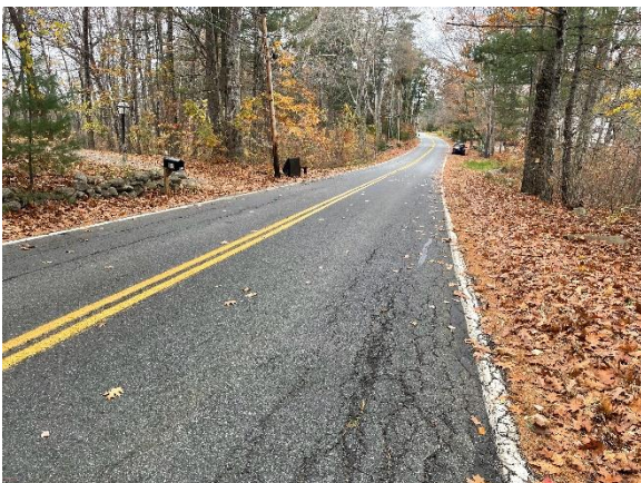
Photo 5: View looking north along Maple Avenue toward the crossing site.
