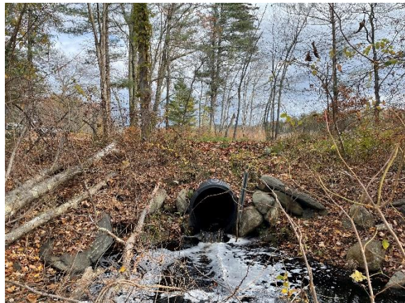
Photo 4: View of downstream culvert outlet, perched \pm 5' , looking east-northeast.
