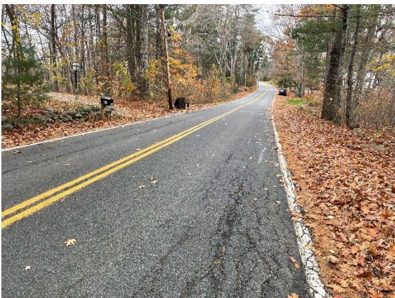
Photo 5: View looking north along Maple Ave toward the crossing site.
